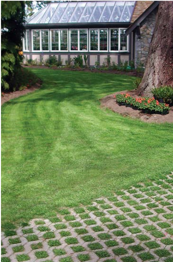
Figure 3. Concrete grid pavements reduce runoff, introduce a cooler microclimate and earn LEED® points.
