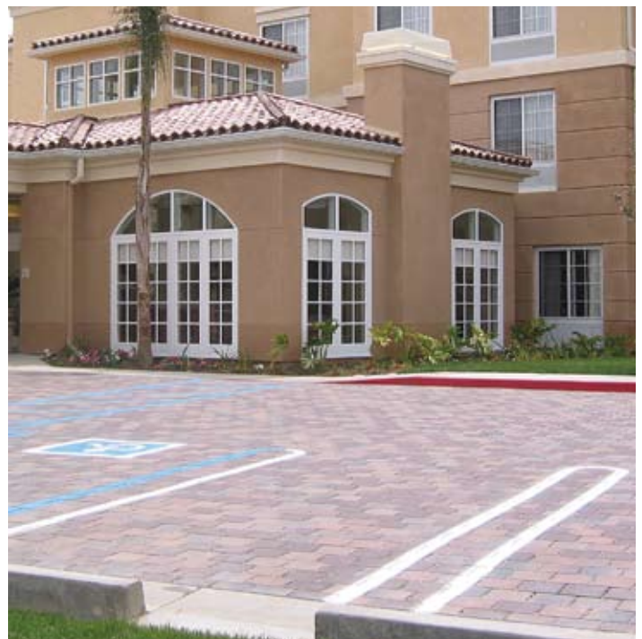
Figures 1 and 2. No matter the climate—wintry Toronto or sunny Southern California—permeable interlocking concrete pavement supports vehicles, reduces runoff and earns LEED® points. The Toronto Harbourfront Fire Station pavement has been in service since 1998.
