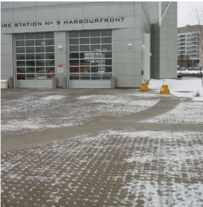
Figures 1 and 2. No matter the climate—wintry Toronto or sunny Southern California—permeable interlocking concrete pavement supports vehicles, reduces runoff and earns LEED® points. The Toronto Harbourfront Fire Station pavement has been in service since 1998.
